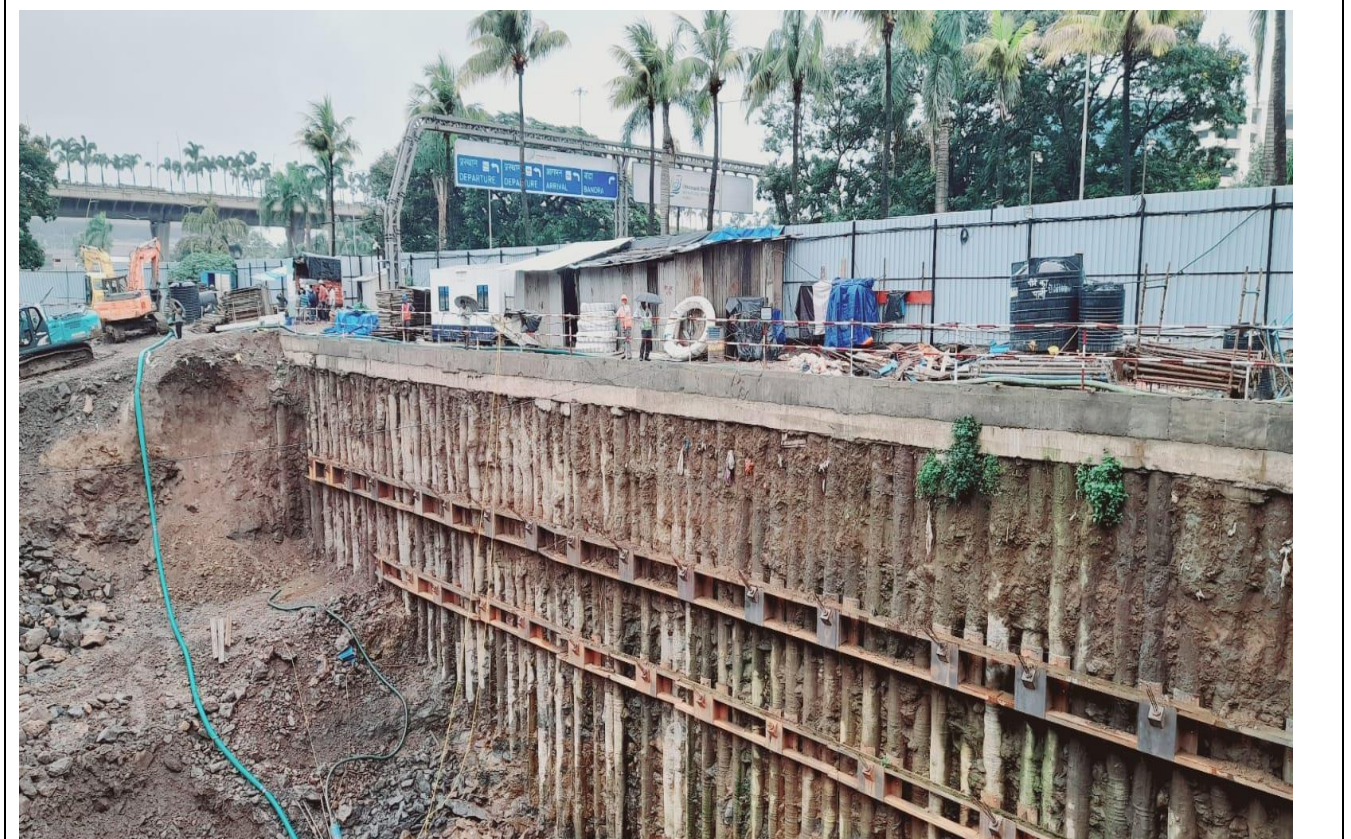
Excavation Process
